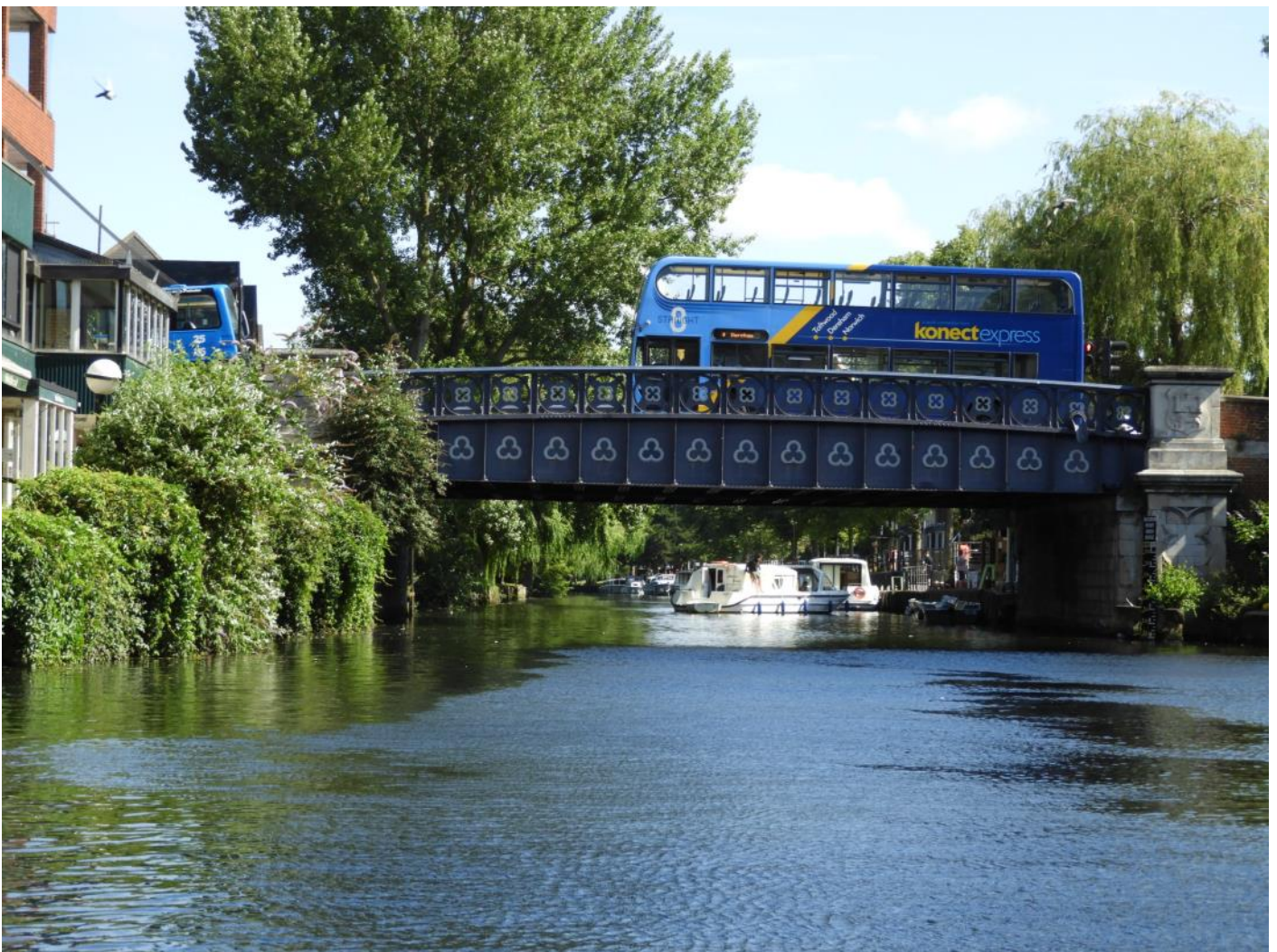
The present Foundry Bridge seen from the river downstream.
